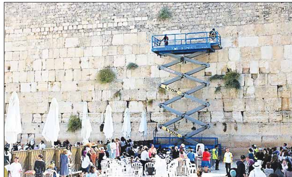
Engineers conduct inspection of the Western Wall
