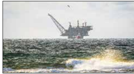
Israeli Leviathan gas field gas processing rig seen from Dor Habonim Beach Nature Reserve
