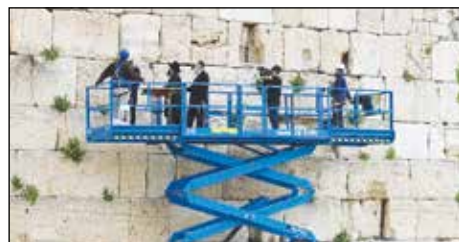
A Western Wall safety inspection on April 3, 2019
